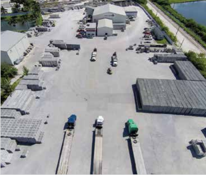
The company's concrete block plant matches the Supermix mission of the 'best product on time'.
