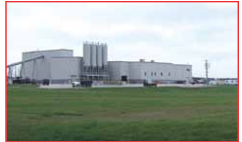
The company spent two years doing extensive site work for Atlas Block's new factory.
